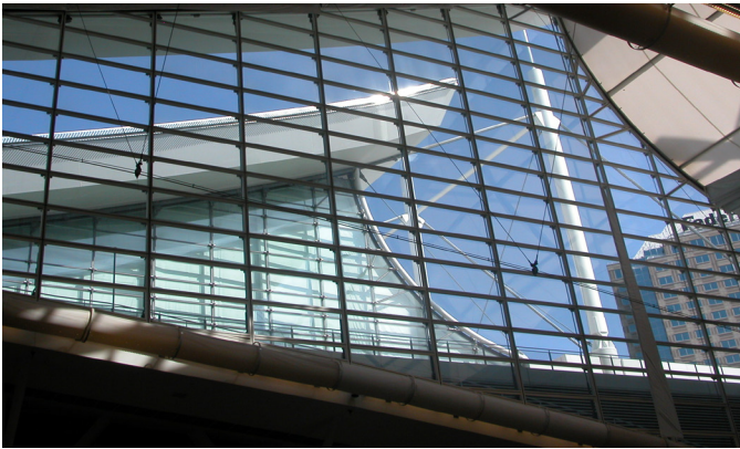
Figure 8. One of the expansive windows bringing light into Halls A, B, and C
