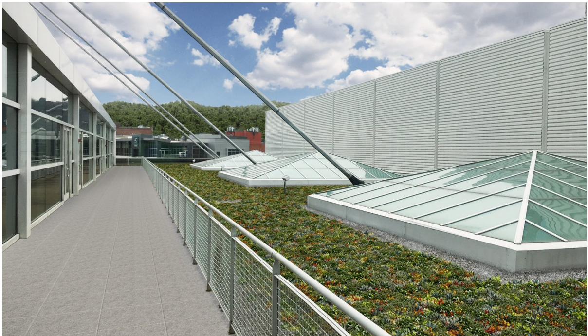
Figure C2. Top: Current ballasted Roof Figure C3. Bottom: Artist Rendering of the new green roof replacement in 2020
